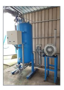
**The AFE Tank Vent Dryer** is available in 3 main configurations to cater to different types and sizes of operation. The system can also be customized according to client's requirements.
